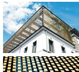
The façade of the Palazzo del Cinema consists of more than forty thousand of gold glistening anodized aluminium flags, which move even in a light breeze. The metallic flags are fixed onto vertical cables. The black stainless-steel cables are pre-stressed in specially made mounting frameworks and the flags attached.
