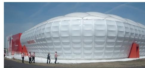
The temporary pavilion belonging to the large Italian Group, Finmeccanica, is to be assembled for 4 weeks every 2 years. The self-supporting steel structure and the two-layer cover have been designed and manufactured for straightforward dismantling and rebuilding.
