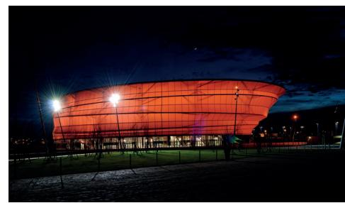
The Zénith is a 'Salle de Spectacle' seating 10.000 spectators situated in the greater Strasbourg area in Eckbolsheim. Five steel rings covered in an orange membrane are poised at different angles and set in a staggered pattern around the massive central oval. [1]
