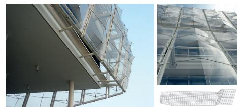
The curtain wall offers protection against superfluous solar energy as it means the shading louvers can be used even in high winds and strong sunshine. The façade consists of 224 panels, each one forming an independent unit. The basis is a rigid frame of hollow sections which is covered by a cable-supported ETFE-foil. [6]
