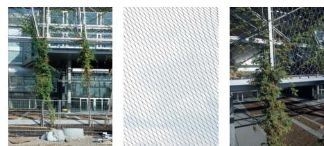
A lattice-style façade for climbing plants, comprising a double layer of stainless steel cable-net, was developed for the SwissRe building. The steel structure, featuring cables and a stainless steel net, was designed for the plants to grow up. [7]
