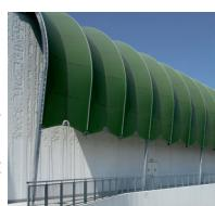
The Italian supermarket chain "bennet" upgrades the façade of its mall with a covering of silicone-coated glassfabric.
