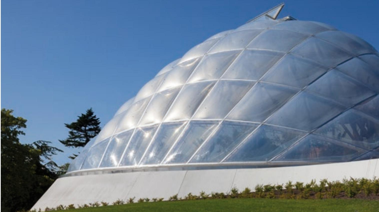
**THE NEW TROPICAL CONSERVATORY** at the Botanical Gardens in Aarhus is like a drop of dew in its green surroundings. Its transparent dome set on an oval base extends the existing greenhouse built in 1969. A special feature of this structure is that it allows for the greatest interior volume with the lowest possible surface area, leading to high energy efficiency. The support structure consists of 10 steel arches, which fan out around a longitudinal and a transverse axis, creating a net of
