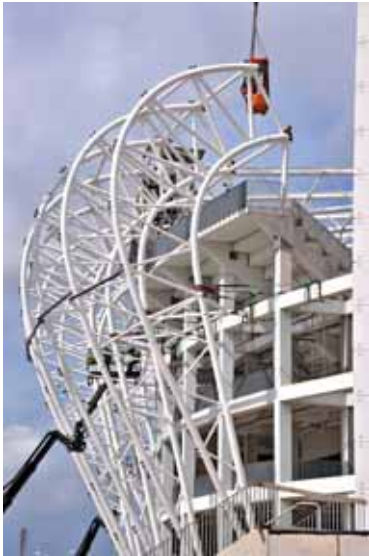
Montage Binderelement © Julius Berger Nigeria Plc
